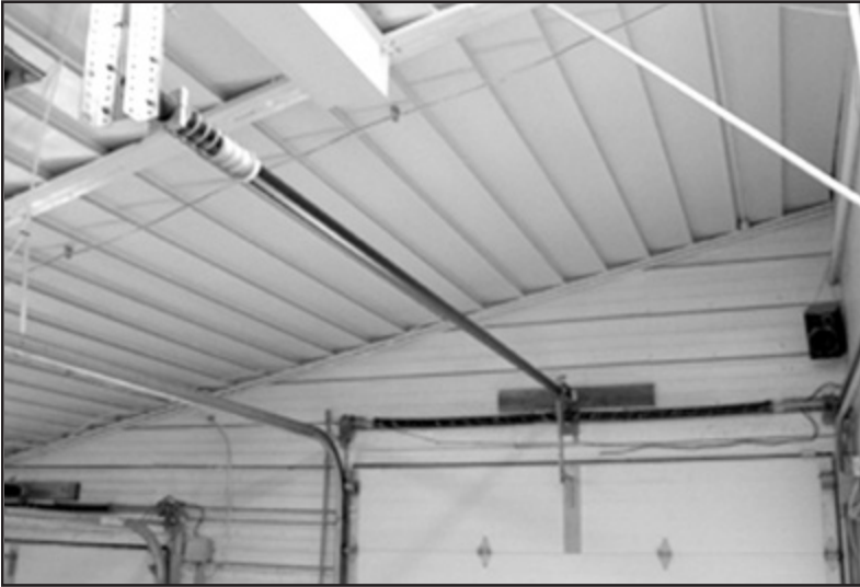
Overview- Installation Complete
