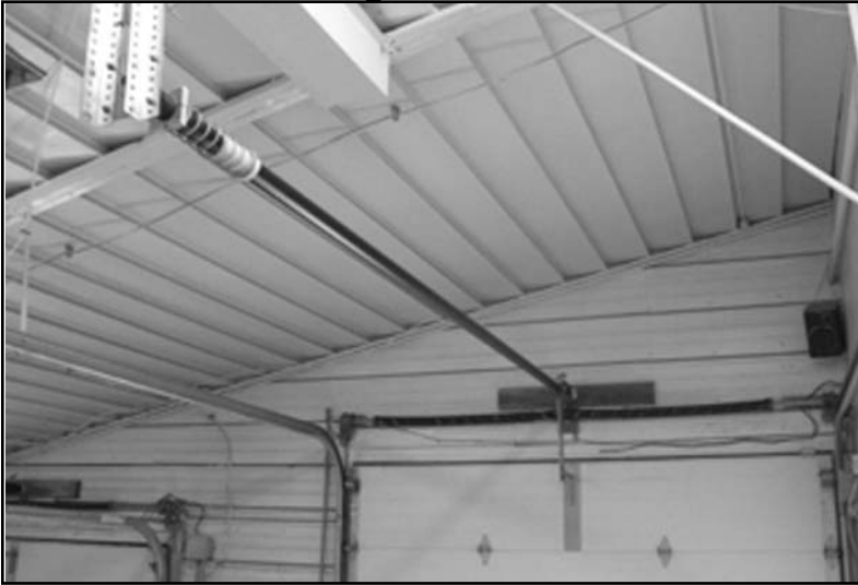
Overview- Installation Complete
